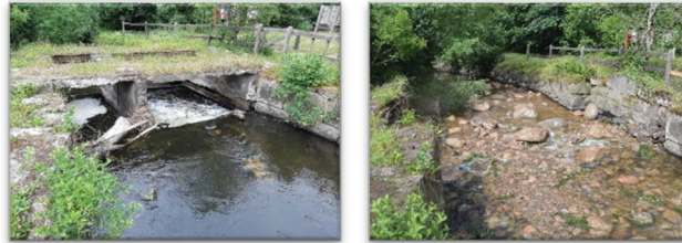
A barrier that has been removed and larger substrate reintroduced into the river. Today fish and other organisms can migrate freely and spawning areas have returned.
